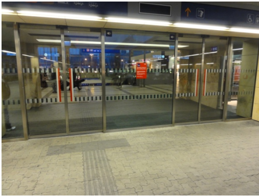
Illustration 50: Well marked glass fronts and sliding doors with marked opening
