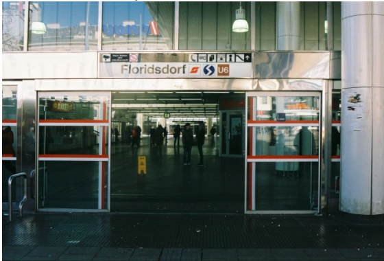
Illustration 36: Well marked door including marking of opening
