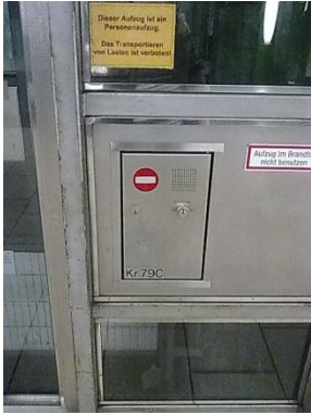
Illustration 37: Lift call-system with hidden call button.
