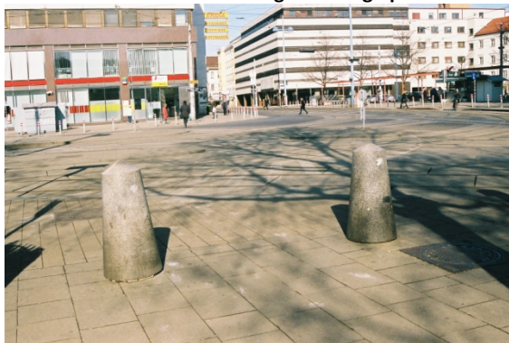
Illustration 42: Non contrasting bollards at half-height
