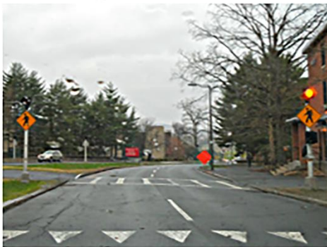
Flashing Signs, Advanced Yield Markings, Rumble Stripes, 1-way Traffic
