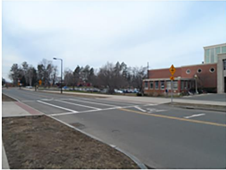
Raised Crosswalk (2 sites)
